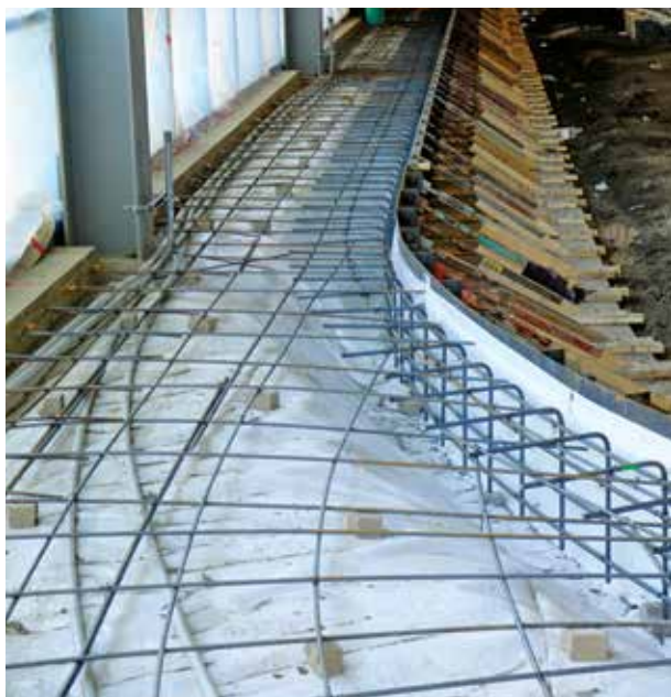
Figure 1. VaporFlex® Standard installation
