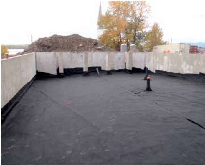
Figure 12. Geomembrane Gas Barrier
